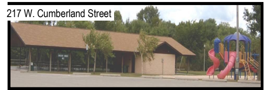
[ ] Shelter house #2 (South) @ Riverside 4 serving tables, 20 regular tables
