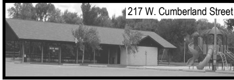
Shelter house #2 (South)
