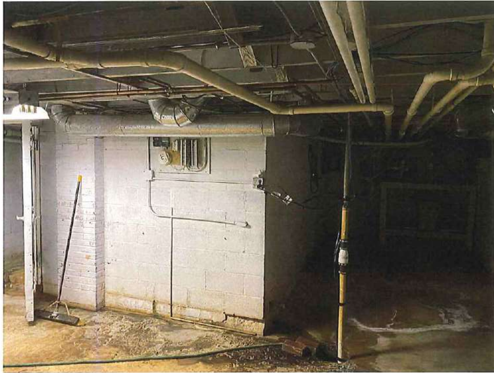
Photo 7: View of basement sump to north. The furnace room is to the left of the sump. (July 7, 2022)
