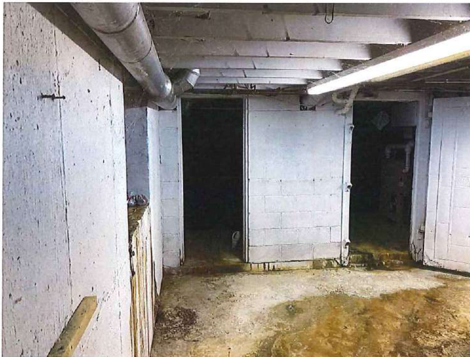
Photo 4: View to north along the western basement wall (closest to Commercial Street) towards water heater / sink room. (July 7, 2022)
