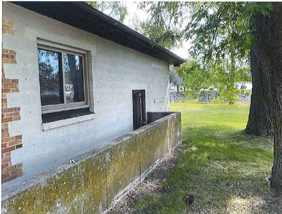
Photo 2: Exterior entrance to the basement of the 120 Commercial Street building. View to northeast. (July 7, 2022)
