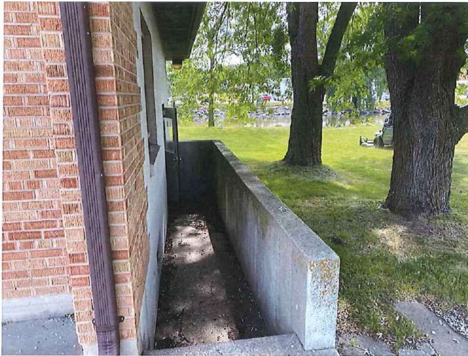
Photo 3: Sidewalk along south side of the 120 Commercial Street building that leads to basement. View to east. (July 7, 2022)
