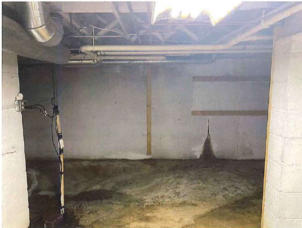
Photo 8: View of sump to east with east basement wall (farthest from Commercial Street) in the background. (July 7, 2022)
