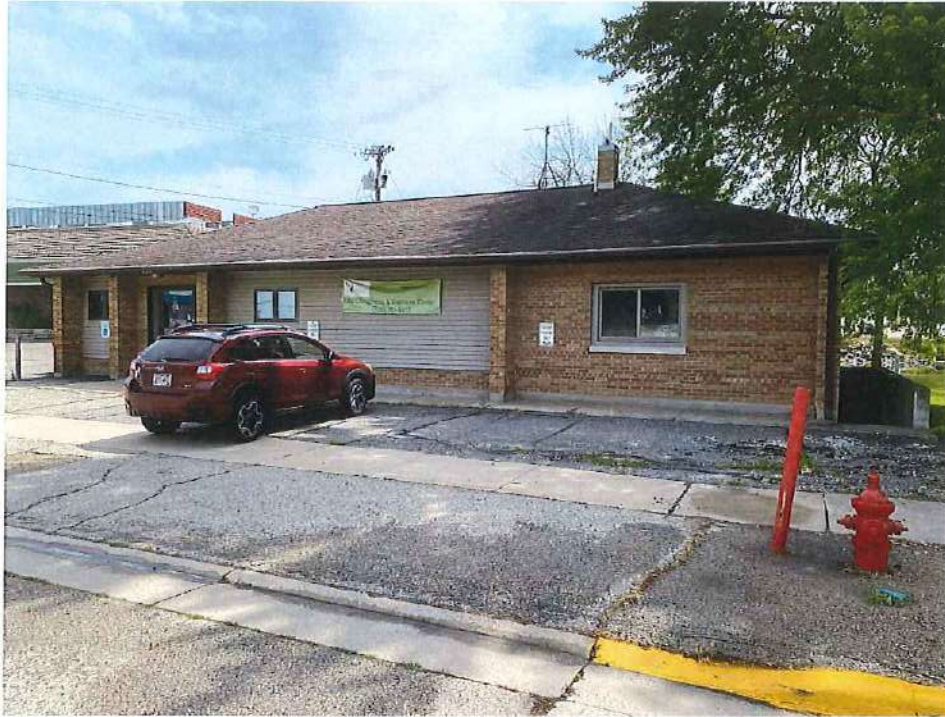
Photo 1: View of the 120 Commercial Street building to the east-northeast. The basement is only present below the south portion of building. (July 7, 2022)
