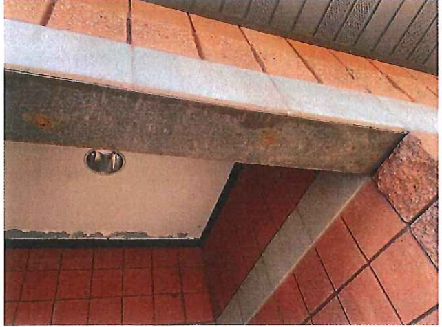
52. CORRODED LINTEL
