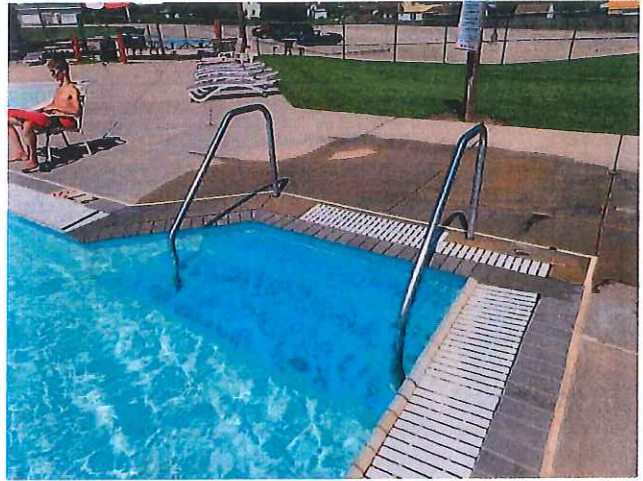
12. WATER OVERFLOWING THE POOL STAIRS
