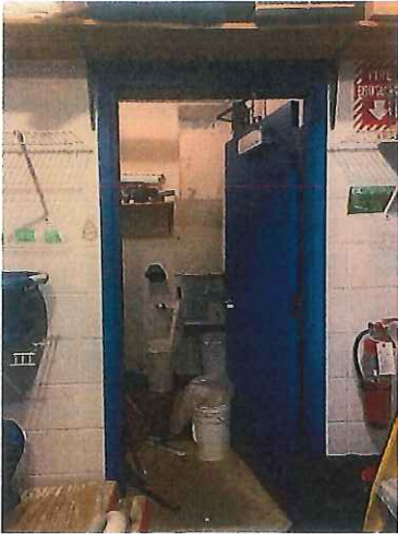
57. MECHANICAL ROOM DOOR
