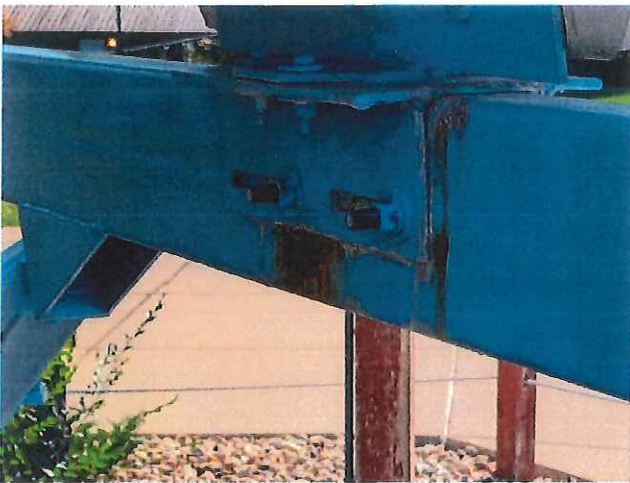
23. SUPPORT CORROSION
