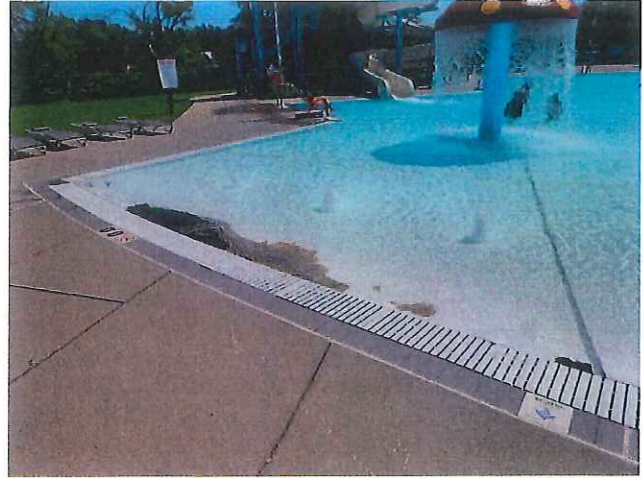
22. FINISH FLAKING OFF IN ZERO DEPTH AREA
