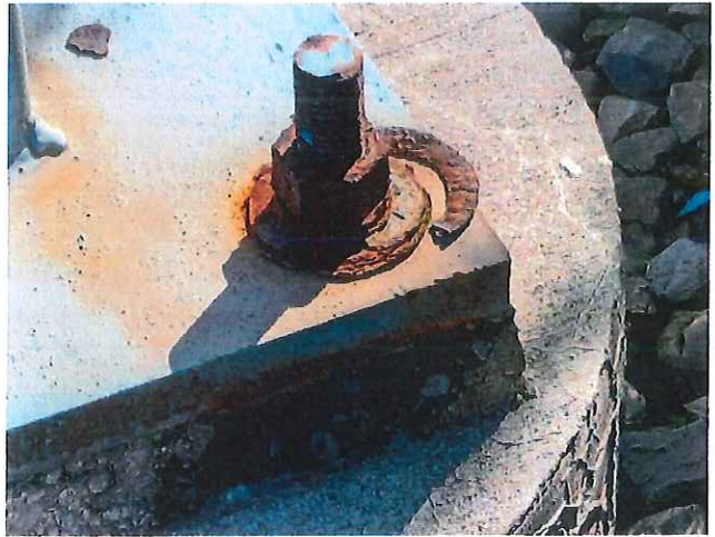
24. CORRODED BOLTS
