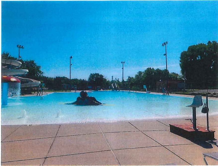
1. OVERALL VIEW OF POOL.
