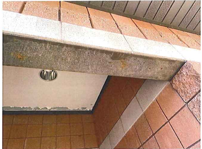
52. CORRODED LINTEL
