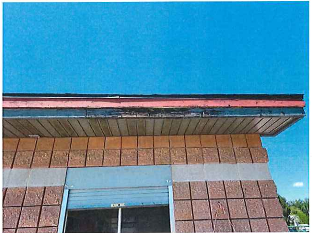
48. WOOD FASCIA BOARD DETERIORATING
