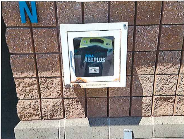
51. CORRODED AED CABINET
