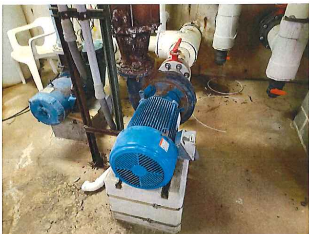
29. CORROSION ON WATERSLIDE PUMP ASSEMBLY
