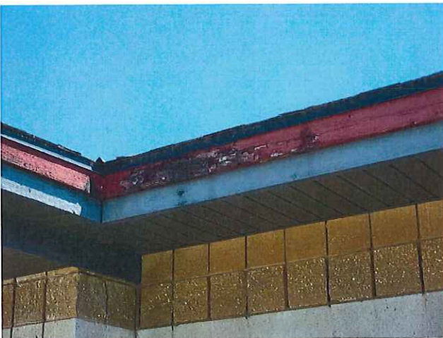
49. WOOD FASCIA BOARD DETERIORATING
