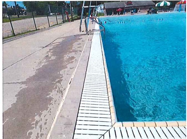
20. NO RIM FLOW OVER GUTTER
