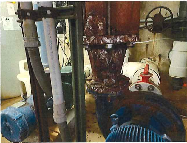
35. HEAVILY CORRODED REDUCER
