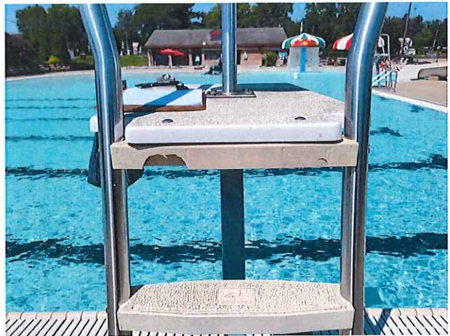
8. BROKEN SUPPORT ON LIFEGUARD CHAIR
