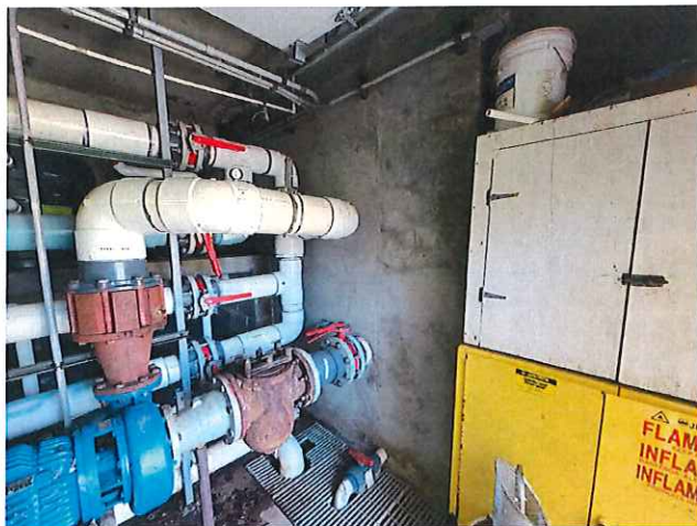
27. SURGE TANK IN MECHANICAL ROOM
