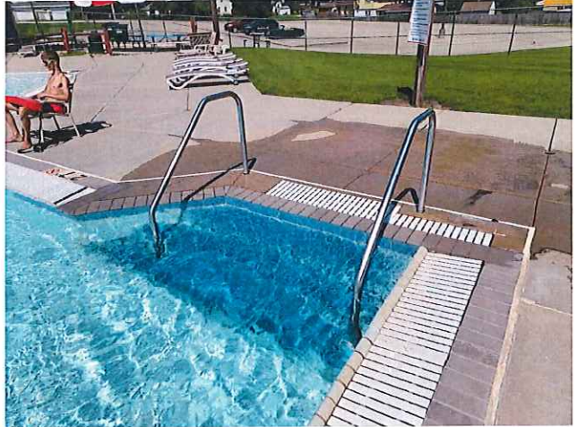
12. WATER OVERFLOWING THE POOL STAIRS
