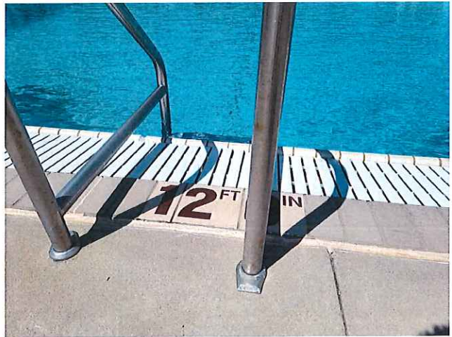
6. CORROSION ON POOL LADDER
