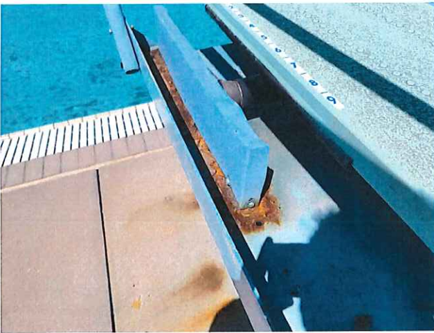
11. CORROSION ON DIVING BOARD ASSEMBLY
