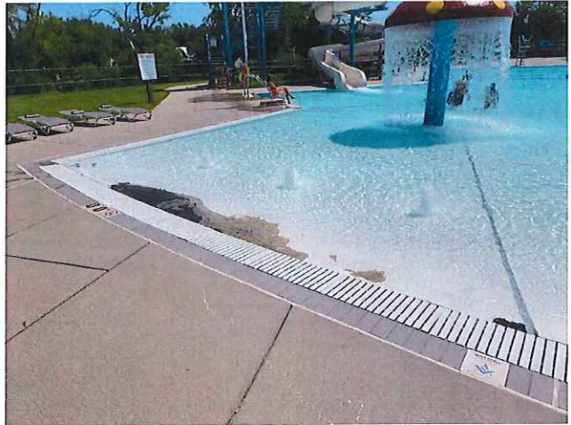
22. FINISH FLAKING OFF IN ZERO DEPTH AREA
