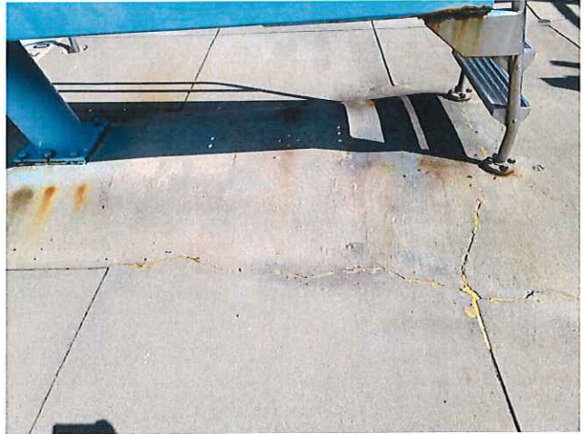
10. CRACKING AROUND DIVING BOARD BASE
