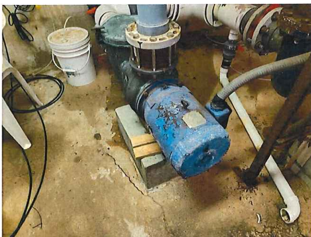
30. CORROSION ON FEATURE PUMP ASSEMBLY
