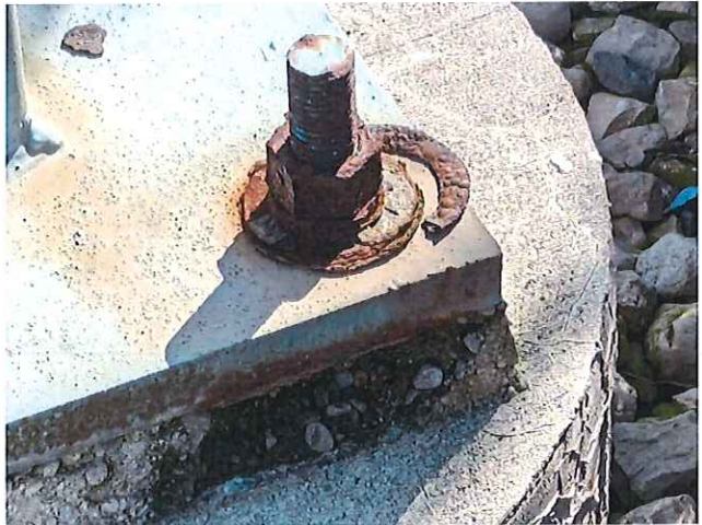
24. CORRODED BOLTS
