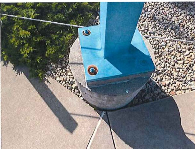
25. EXPOSED FASTENERS OUTSIDE OF BARRIER
