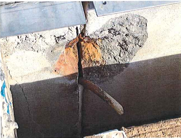
13. BROKEN GUTTER JOINT
