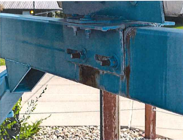
23. SUPPORT CORROSION
