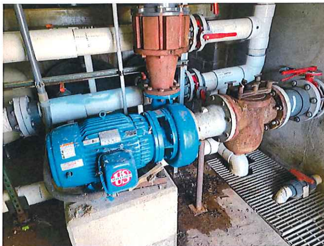
28. CORROSION ON RECIRCULATION PUMP ASSEMBLY
