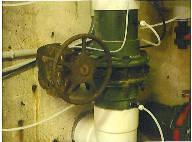
34. CORRODED VALVE
