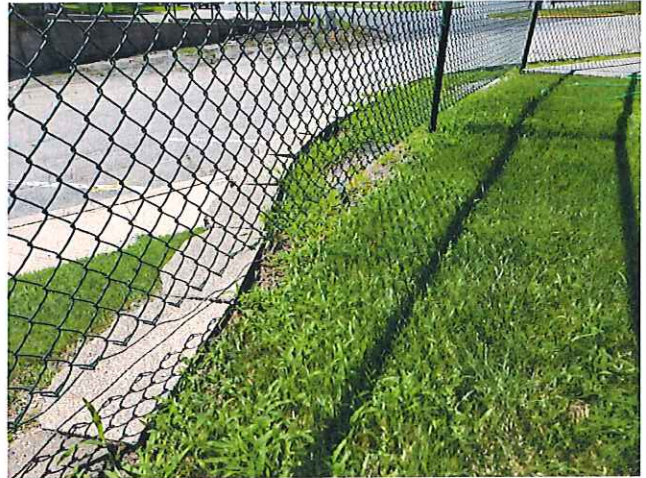
16. GAP UNDER FENCING LARGER THEN 4"
