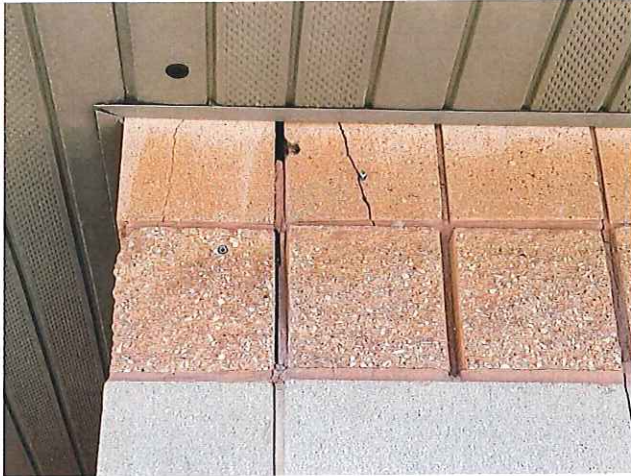
39. CRACKS AND SEPARATION OF CMU
