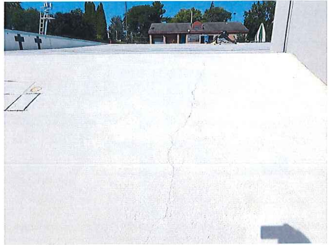
18. CRACK ON TRANSITION PANEL
