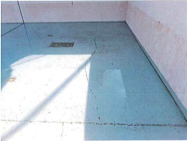
17. CRACK IN DIVING HOPPER
