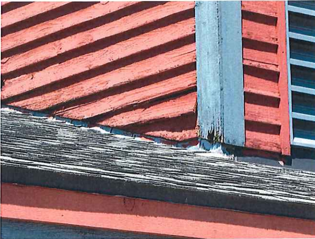
45. WOOD SIDING DETERIORATING
