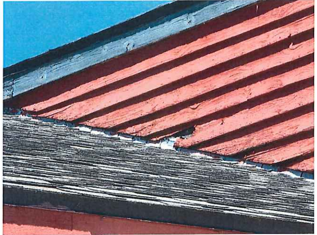
46. WOOD SIDING DETERIORATING
