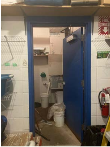
57. MECHANICAL ROOM DOOR
