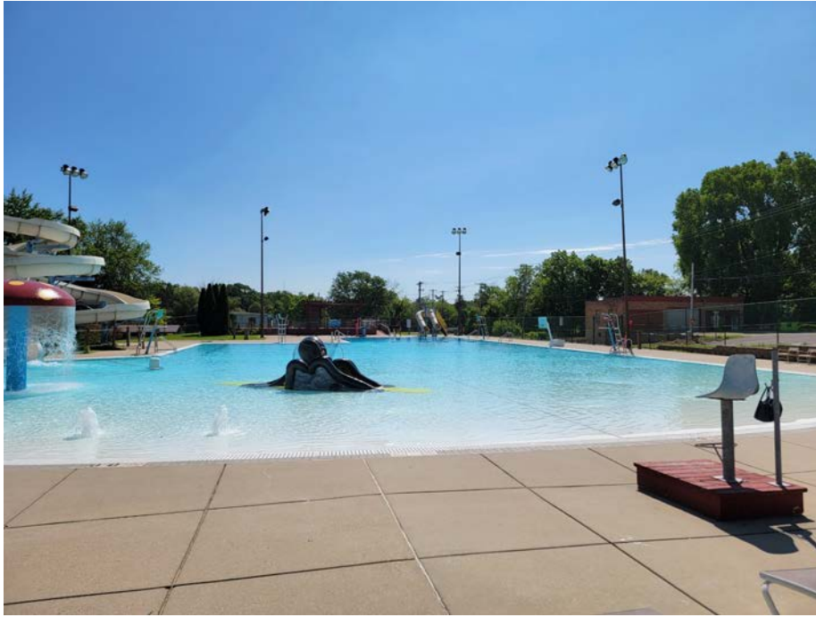
1. OVERALL VIEW OF POOL.
