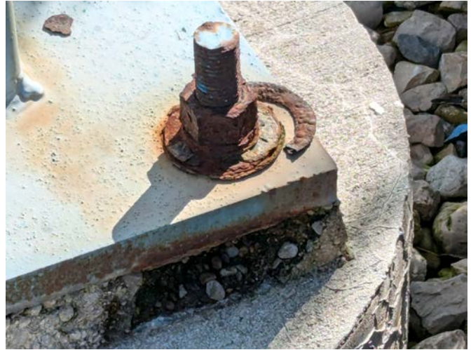
24. CORRODED BOLTS
