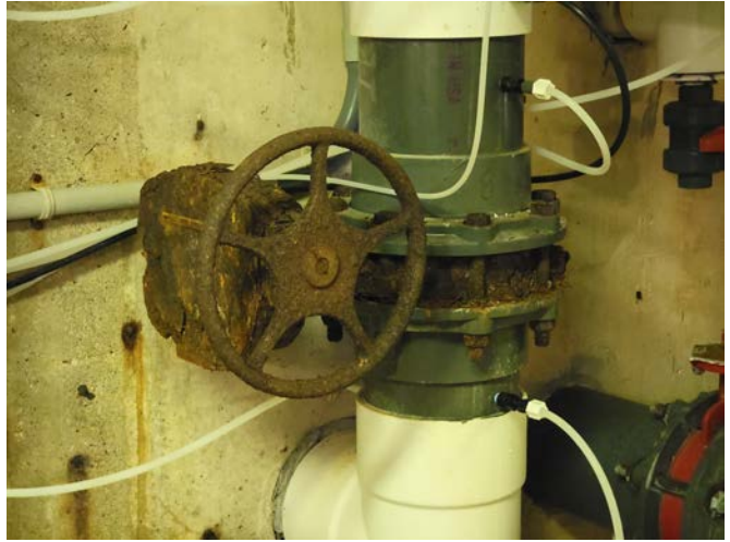
34. CORRODED VALVE
