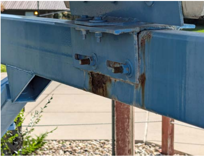
23. SUPPORT CORROSION
