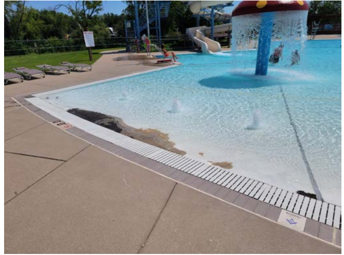
22. FINISH FLAKING OFF IN ZERO DEPTH AREA
