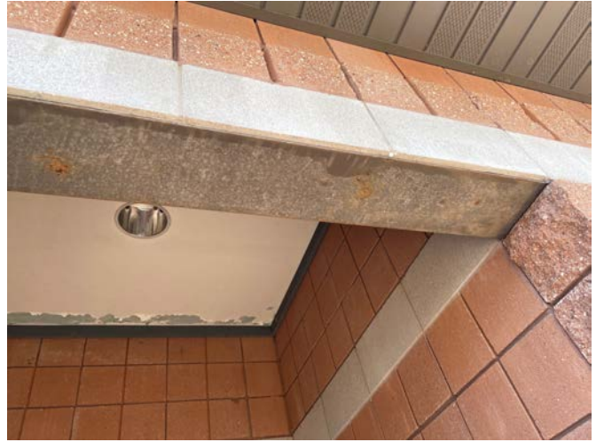
52. CORRODED LINTEL
