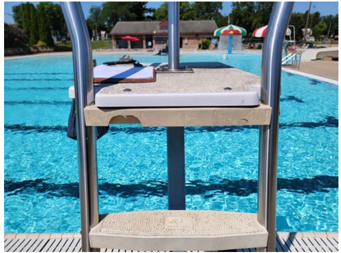
8. BROKEN SUPPORT ON LIFEGUARD CHAIR
