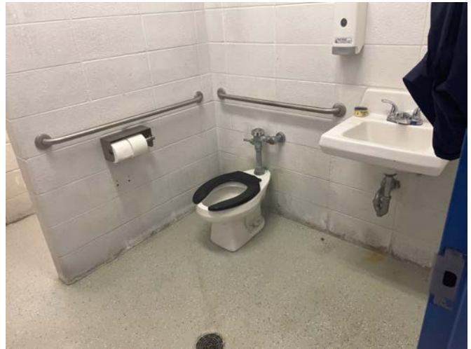
68. MEN'S STAFF RESTROOM
