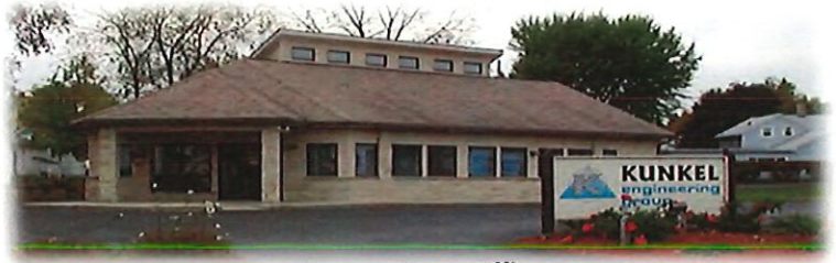
Beaver Dam Office
